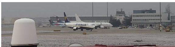
10 EHF Radar installations
